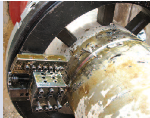
Cold cutting of a pipeline
