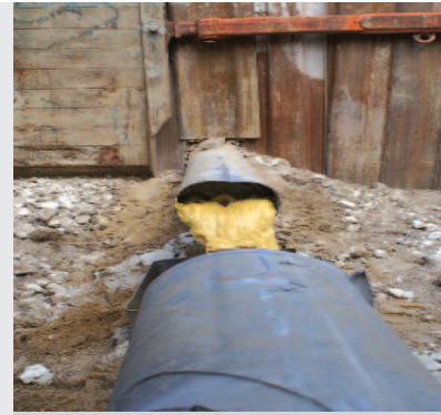
Damaged pipeline
