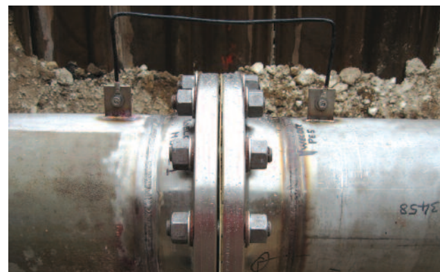
Repaired pipeline with cathodic protection system
