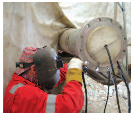
On-site pipe welding
