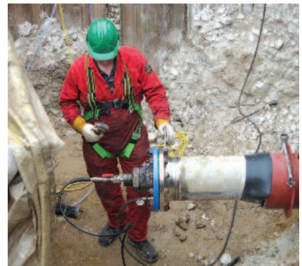
Hydrotesting of flange weld joint
