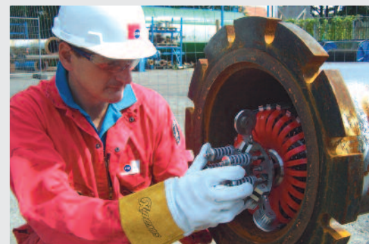
PECAT® being positioned in pipeline
