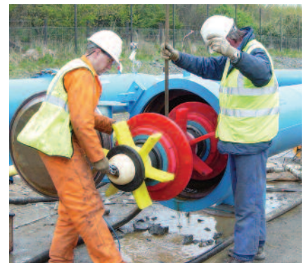
Test loop and testing of dual-diameter cleaning tools
